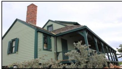
Gilbert's Bar House of Refuge, Hutchinson Island
